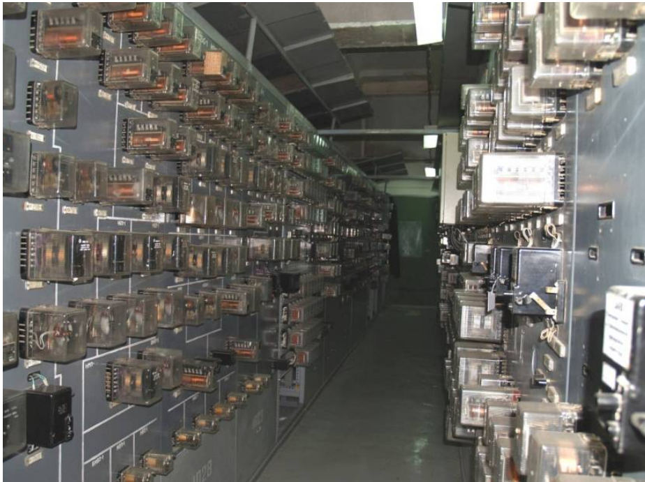
Logic solver (relay-based I&C of VVER type reactor)
